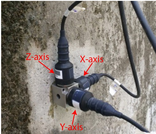
Figure 2: Three single-axis accelerometers will be attached to the wall.
